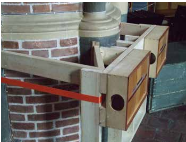
Tie-down belts used to anchor to columns
