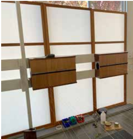
Wall-mounted Cheapest and easiest method using 2x6s (5x15s) and screws
