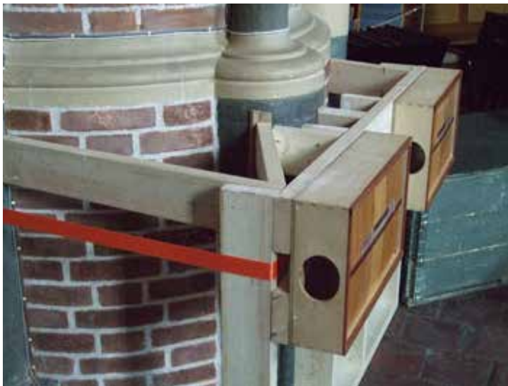
Tie-down belts used to anchor to columns
